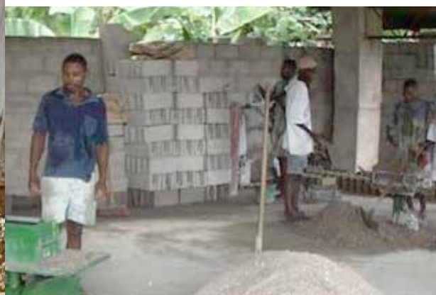
Haiti [Camp Perrin] : making concrete blocks.
